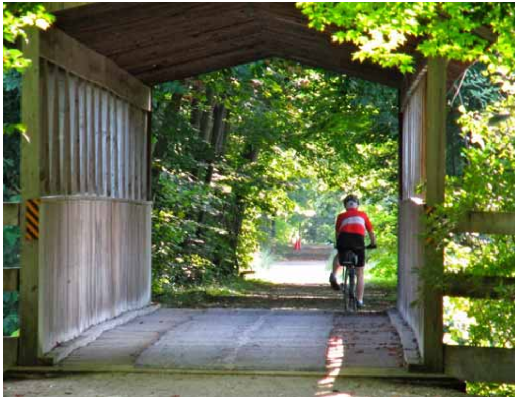
The Michigan Department of Natural Resources is replacing the Donald F. Nichols Covered Bridge over the Black River on the Kal-Haven Trail.
