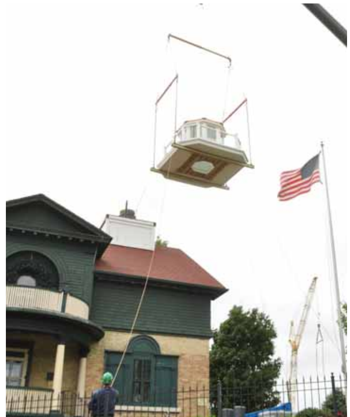
The archival photo taken Sept. 30, 2014, shows the new lantern room installation. Photo provided by Josh McIntyre.
