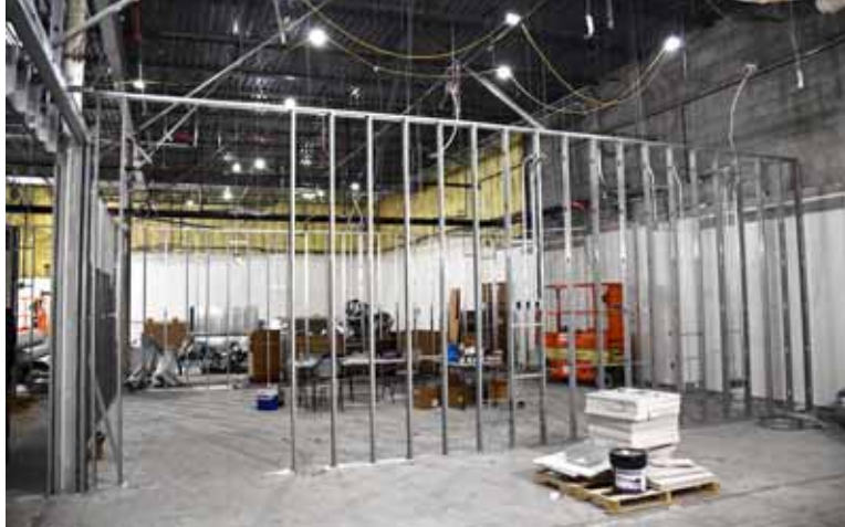
The initial stages of construction in the new facility at 1001 U.S. 20.
