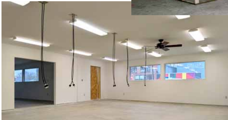
These provided photos reveal the work being done at the 116 Building.
