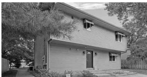
204 WASHINGTON PARK BLVD, MICHIGAN CITY 4 BED / 4 BATH • 1,836 SF
